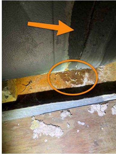
Furnace and evaporator located in attic
