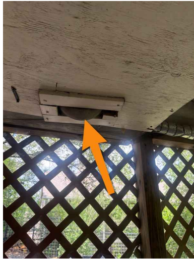
Under pier and beam elevated section
