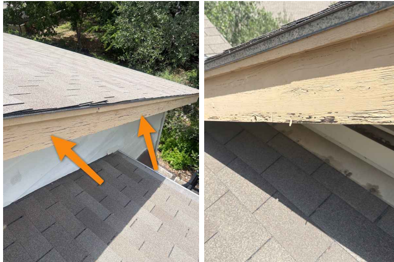
Above roof level on fascia board
