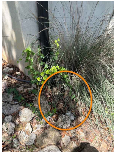
Front Right Corner Of Home
