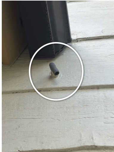
Secondary Condensate Drain at Back Of Home
