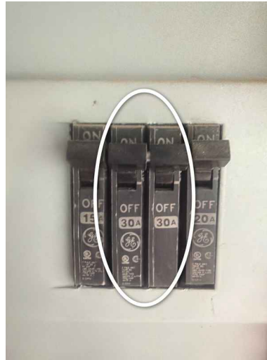
30 amp circuit breaker installed
